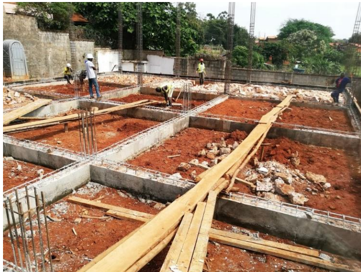
Casting the beams and Levelling the ground with type 1 hardcore
