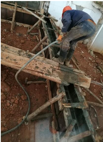
Casting the beams and Levelling the ground with type 1 hardcore
