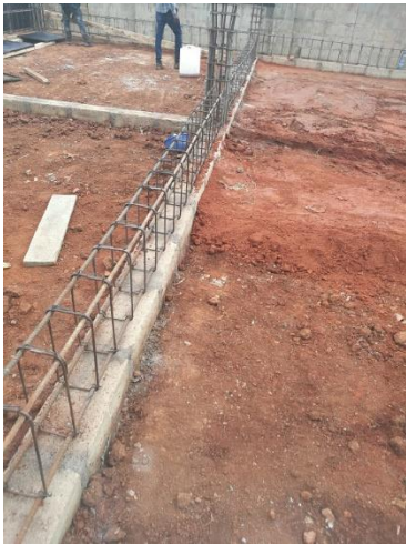
Casting the beams and Levelling the ground with type 1 hardcore
